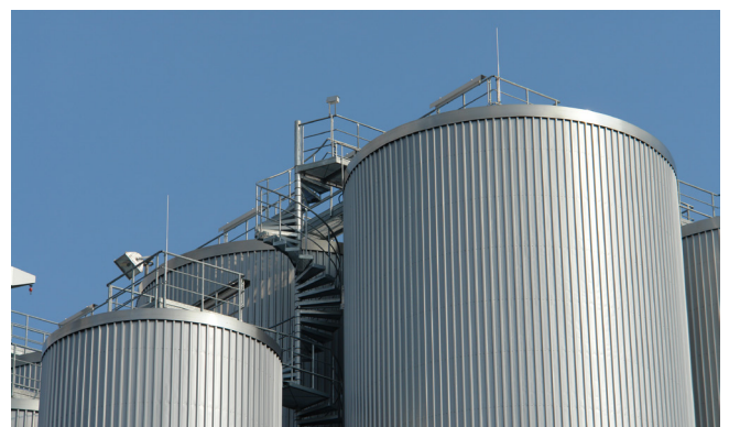
Figure 2: ...cylindro-conical tanks have the advantage that the contamination risk is almost zero
