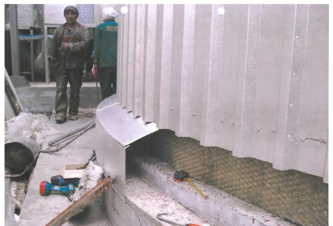
Figure 8: The area between the tank base and the start of insulation must be considered on-site
