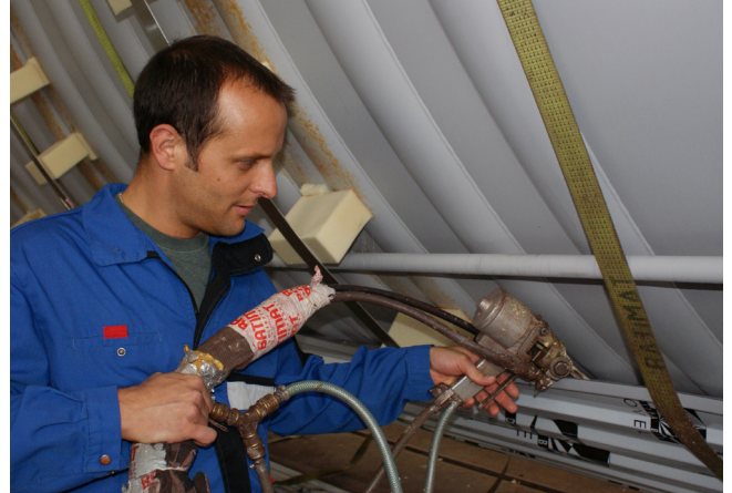
Figure 6: A CCT is insulated
